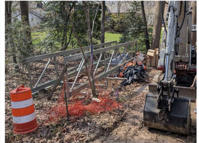
Partially assembled bridge ready for placement
