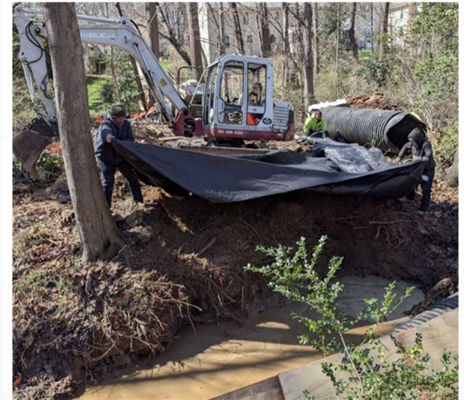
Placement of filter fabric on bank
