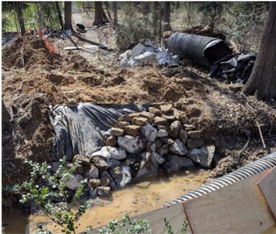
Protective rip rap on top of Fabric underway
