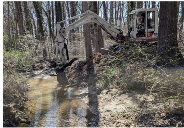
Excavation of stream bank
